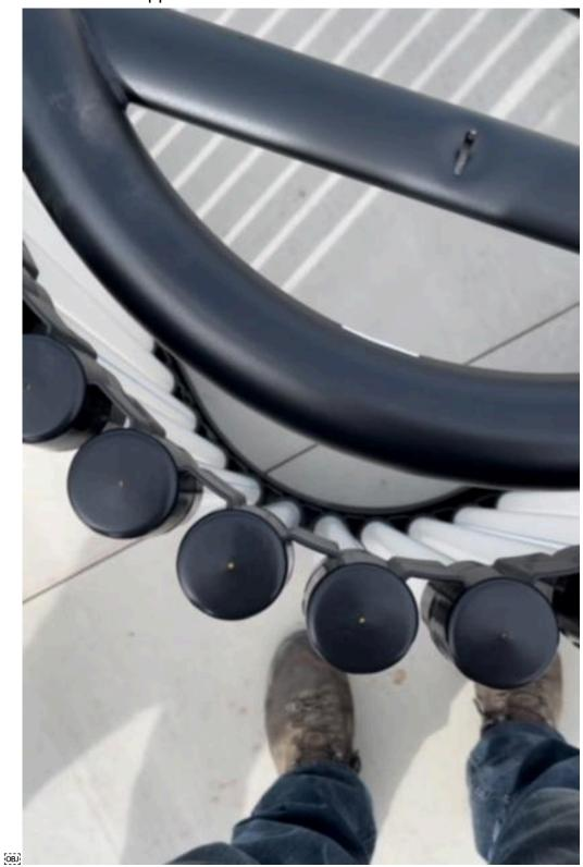
Step 4. At each corner, cut the black ribbing between the black caps so that the pipes will move closer together. Cut in 5 or 6 places between every other pipe.
